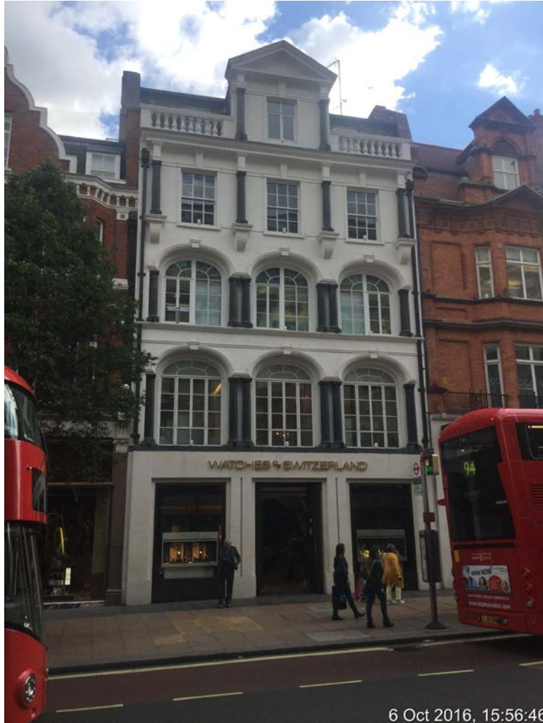
Oxford Street Frontage (Top) and North Row entrance to upper floors (Bottom)
